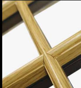
In order to meet modern building regulations and because we are not constrained by glass technology of the period, Residence 9 is made from complete pieces of glass where glazing bars are clad to the glass rather than making individual, small glass units. Internal spacer bars give the appearance of individual units, with the performance of a single, larger sealed unit.
